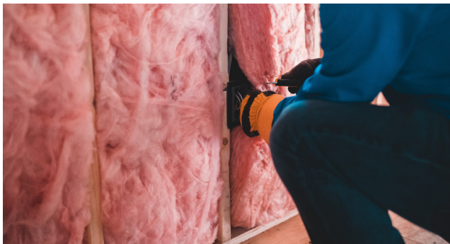
ABOVE A contractor works with insulation
